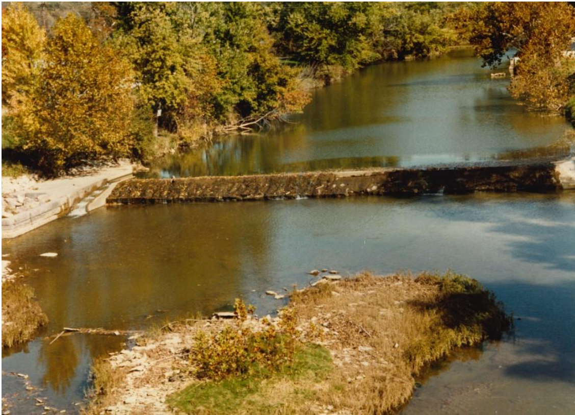
Low Head Dam #1 Built in 1930's
