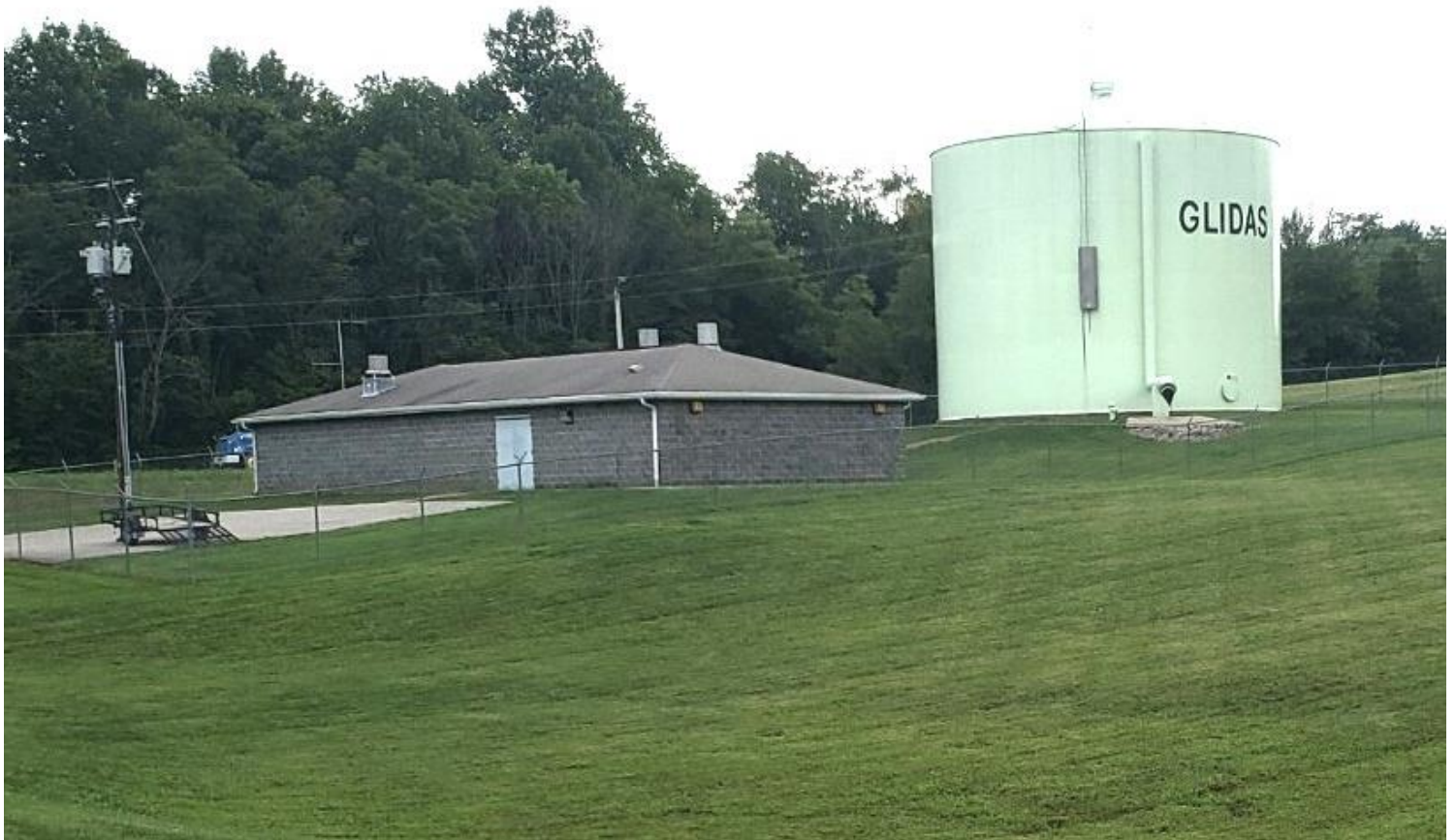
Glidas 500,000 Gallon Tank & Booster – Built 1999.
