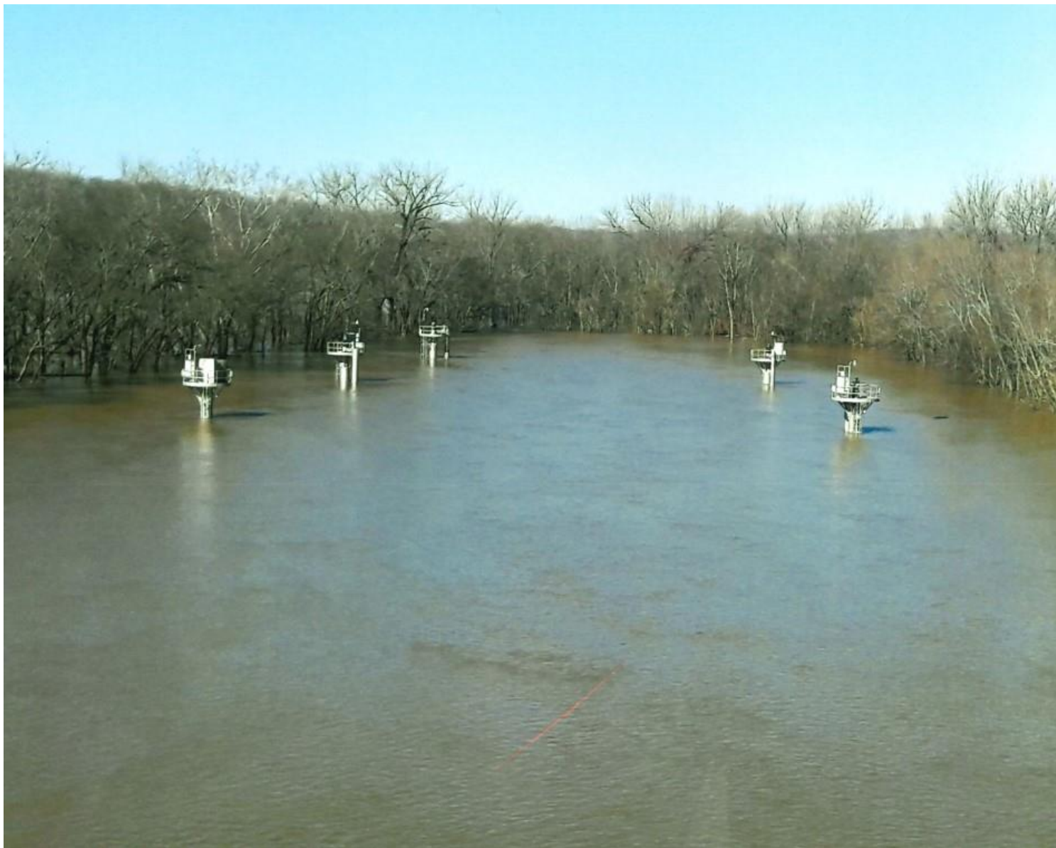
Corydon's Five Wells Along the Ohio River During High Water Conditions. They are Elevated for This Reason.
