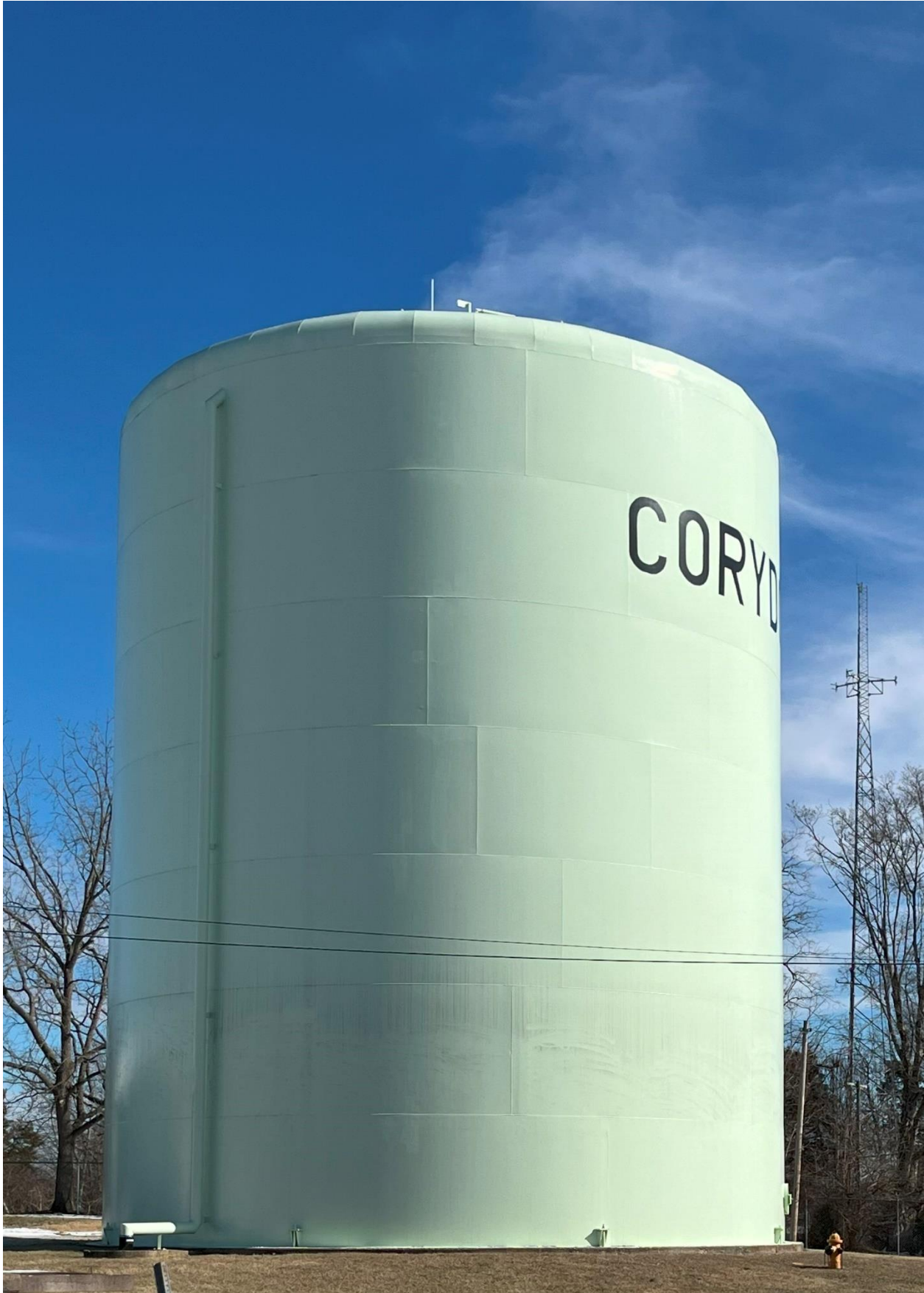
778,000 Gallon East Storage Tank – Built 1984
