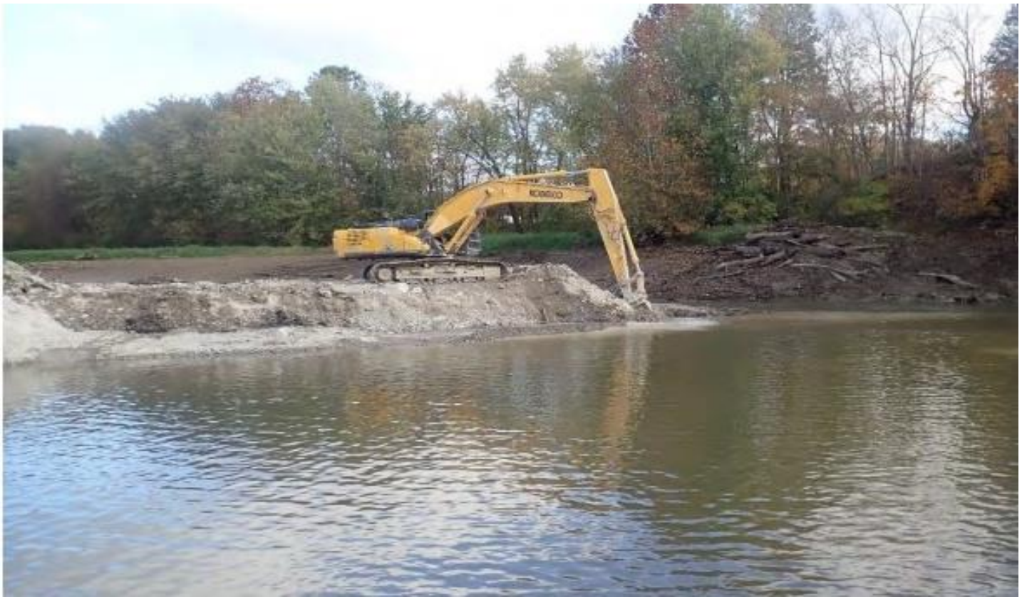
Dam #3 Removal – October 2019
