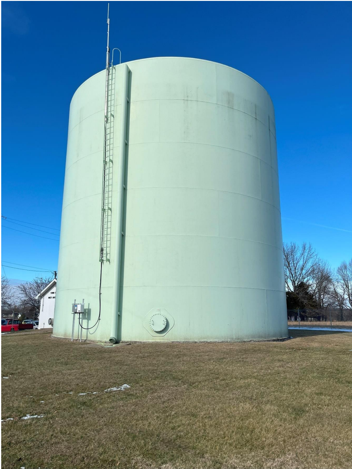
West 500,000 Gallon Storage Tank – Built 1966
