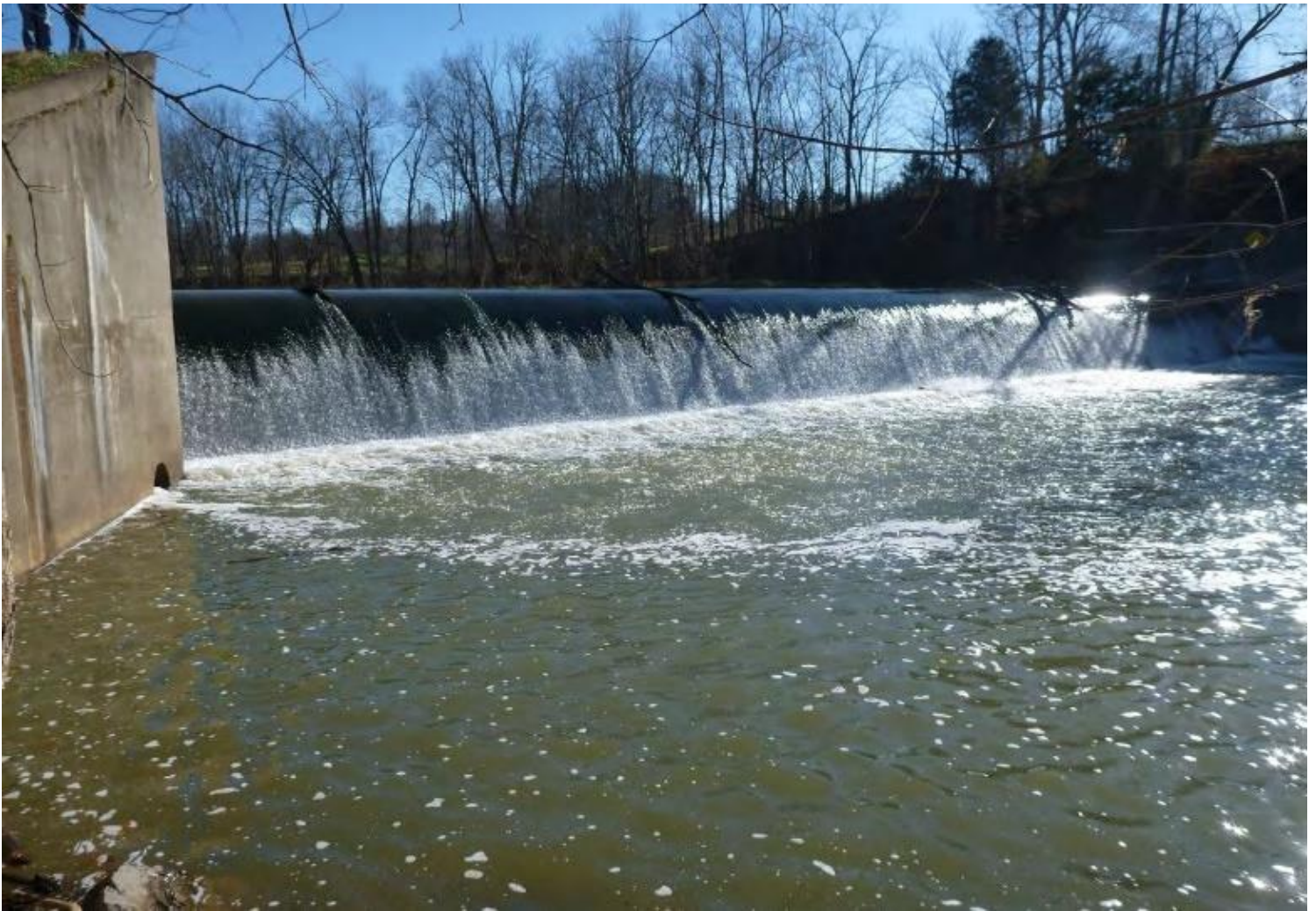
Low Head Dam #3 Built in 1957
