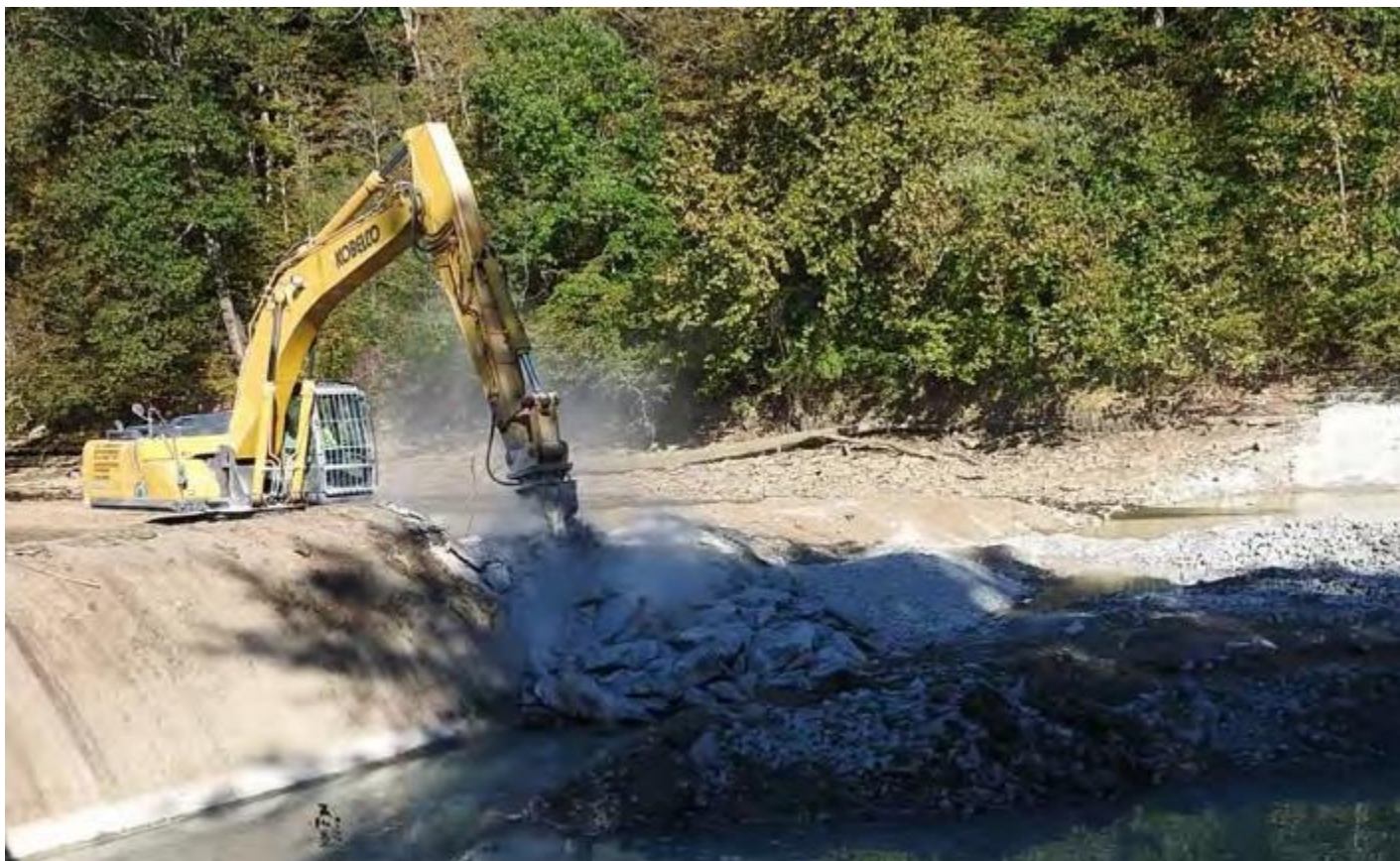
Dam #2 Removal – October 2019
