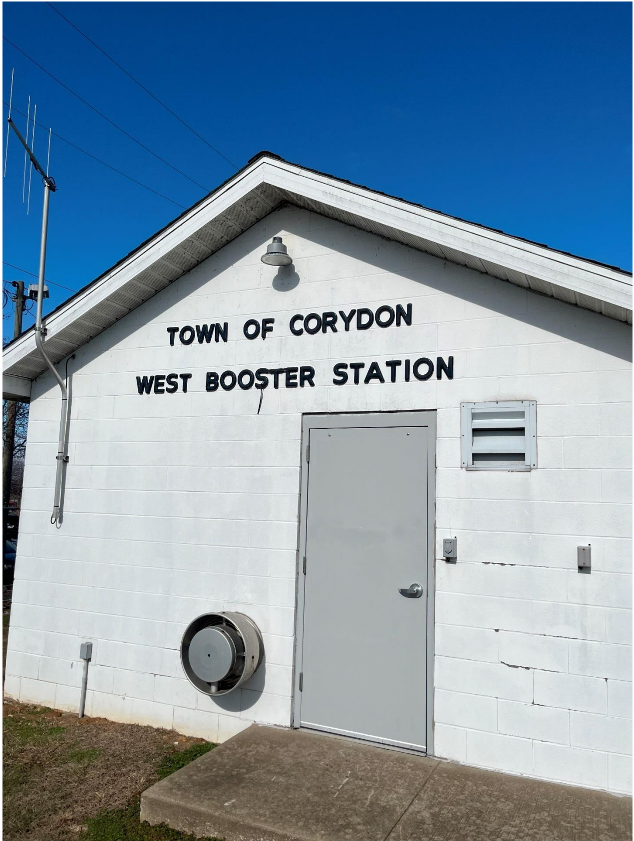
West Booster Station - Exterior
