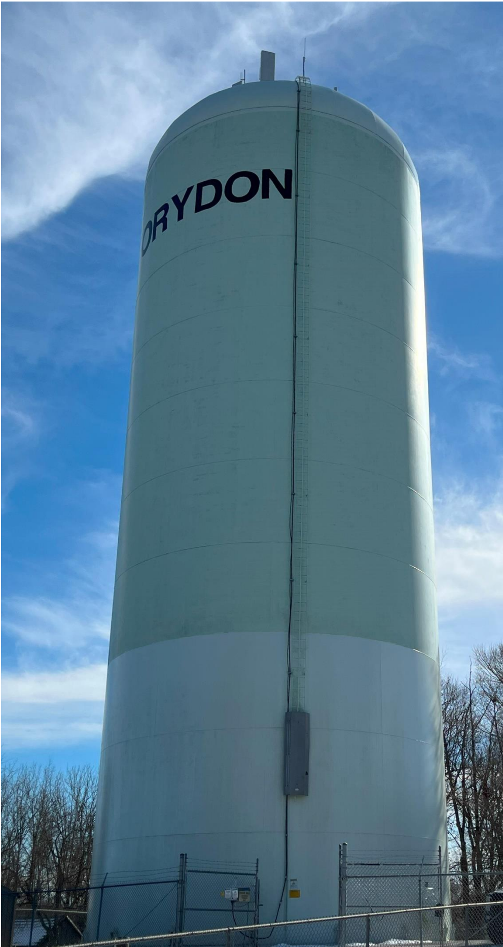
South 968,000 Gallon Storage Tank – Built 1992
