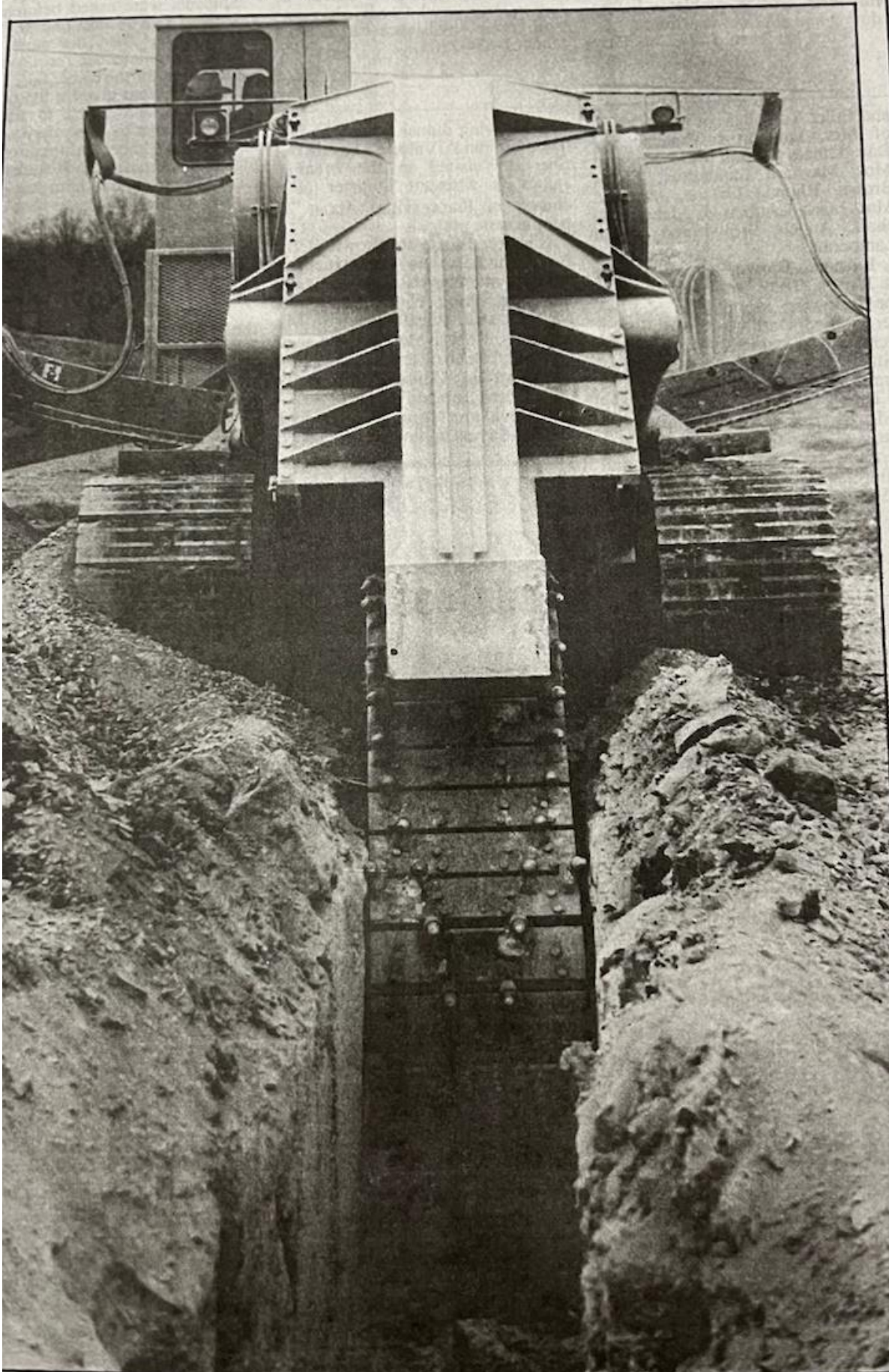
Rock Trencher Opening Ditch for 18" Water Main - 1992
