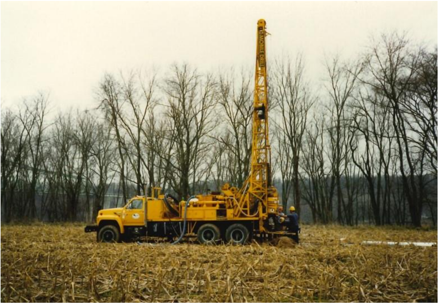
Test Well Being Dug at Mauckport - 1991
