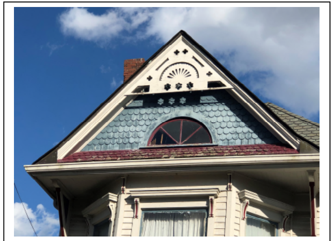
The fishscale shingles and gable ornament are key elements of the architectural character of this Farquar Avenue home.
