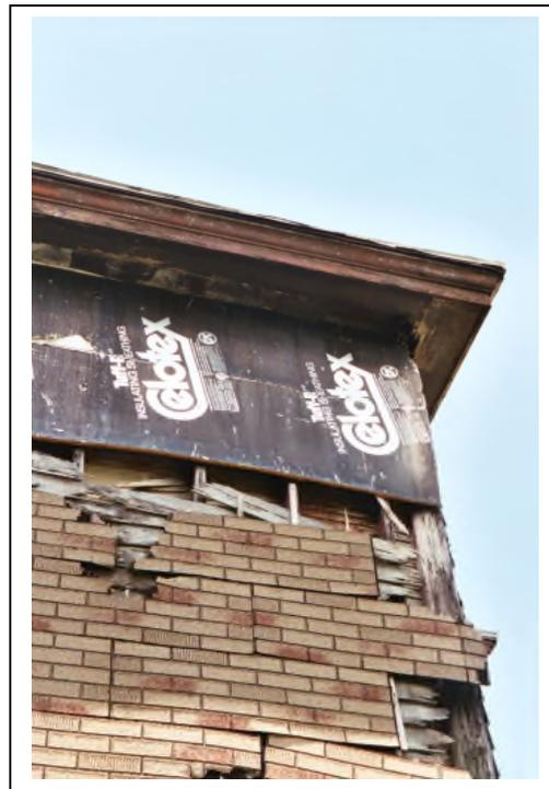
*Water can be the worst enemy of a building if not properly controlled. Leaking box gutters and lack of downspouts caused significant damage to the siding and structure of this New Albany home.*
