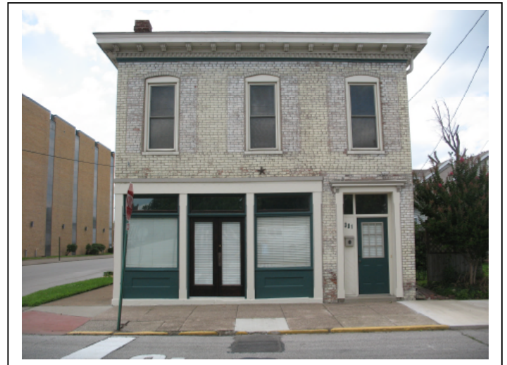
Although it now is used as a residence, retention of the original, paired front doors helps maintain the historic character of this neighborhood commercial building in Jeffersonville.
