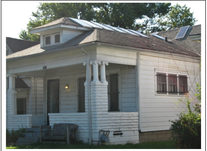
The solar panels in the above example should have been installed in a much less conspicuous location. The tangle of wires leading down from the panels is also not consistent with these design guidelines. The panels on the Nashville, Indiana church below are much more appropriately installed and are almost invisible at street level.
