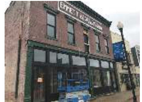
Beanblossom Building Progress
